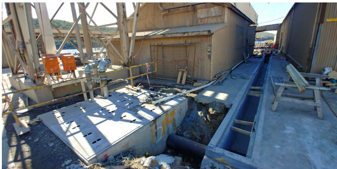
Figure 2-8 Image of one of the stormwater pits, and drains installed at the Wharf
